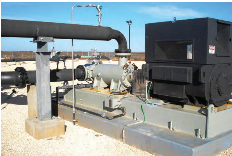
The simple design of the three screw pump (just three rotating parts and one shaft seal) offers advantages for a variety of industries and applications.
