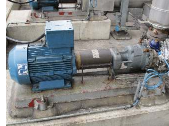
Magnetically-coupled centrifugal pump of the CNH-ML series providing column circulation (liquid: naphtha)
