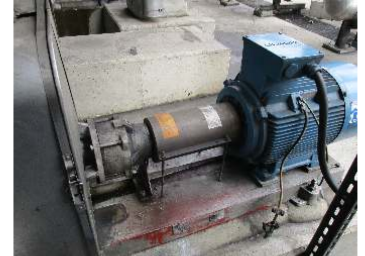
Centrifugal pump of the CTWH series providing column circulation (liquid: base oil)
