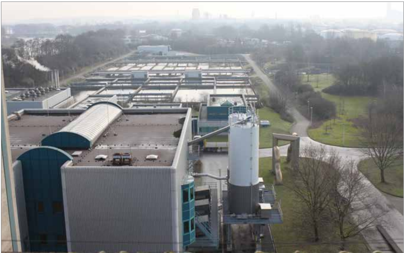
Figure 1: Plant showing sludge silos.
