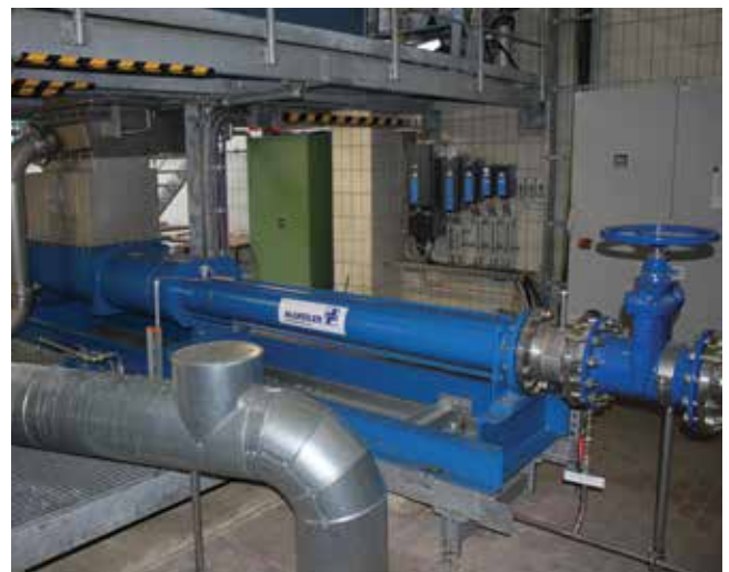
Figure 4: Four-stage solid-substance progressive cavity pump, used as a residual sludge discharge pump below the centrifuge.
