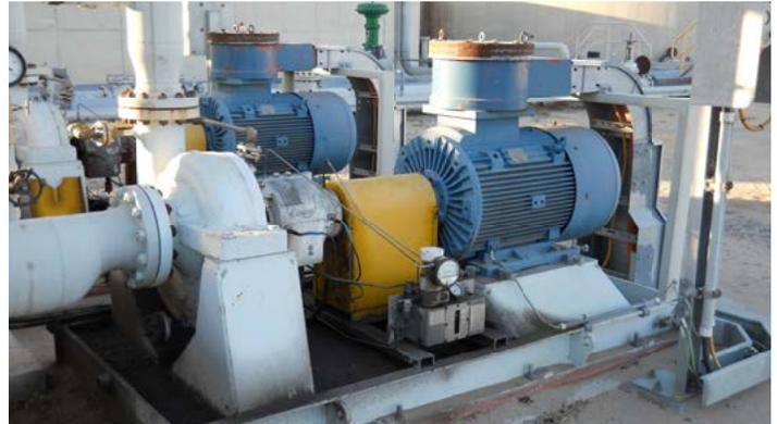
*LubriMist® supplying oil mist lubrication to Tank Farm Pump in Australian Refinery.*
